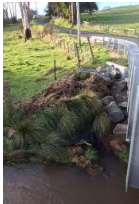
Section of roadside verge adjacent to the river on Paradise Road. This was covered with weed gunnel and planted out with native sedges to reduce the need for weed spraying as part of road maintenance, therefore reducing chemicals entering the watercourse.
