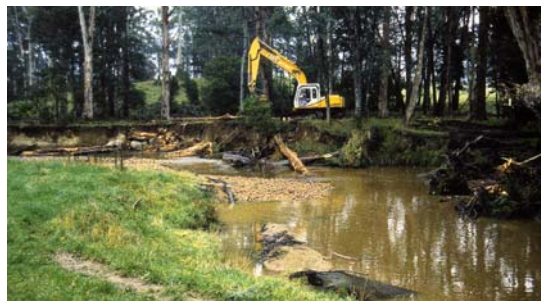
Adding woody debris to the Dasher River
